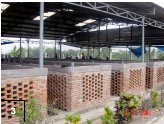
Photo 1, 2 & 3: 3 (three) ton/day capacity community based compost plant located at located at Nhon phu Ward of Binh Dinh Province of Quy Nhon City, Vietnam. Photo 4: Compost plant managers explaining the operation of compost plant to the international participants.
