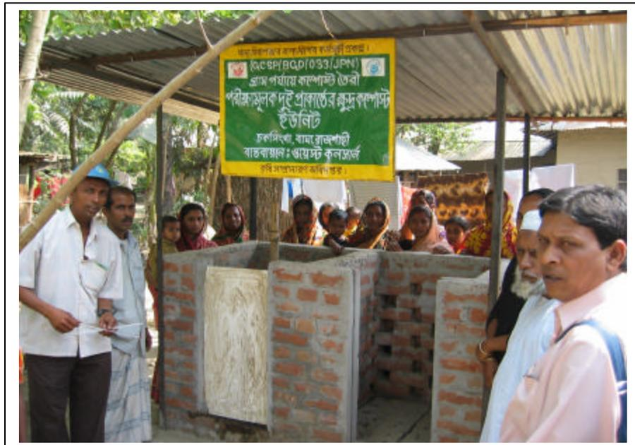
Twin box type composting system using brick masonry introduced by Waste Concern at Chak Singa, Bagha, Rajshahi
