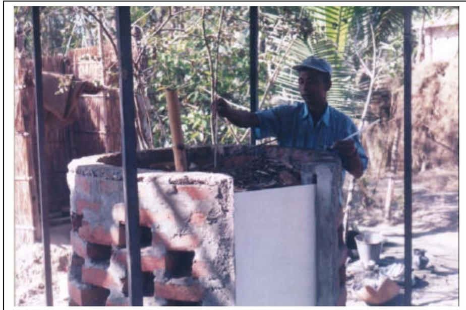
Circular shaped compost box using brick masonry used for compost production designed by Waste Concern at Chak Singa, Bagha, Rajshahi
