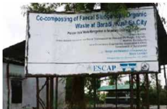
Figure 10: Co-Compost Plant at Baradi
