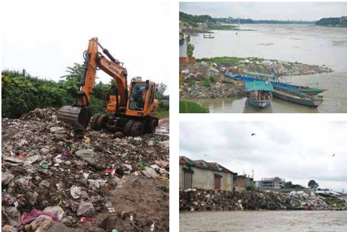
Figure 11: Dumping Site for Generated Solid Waste
