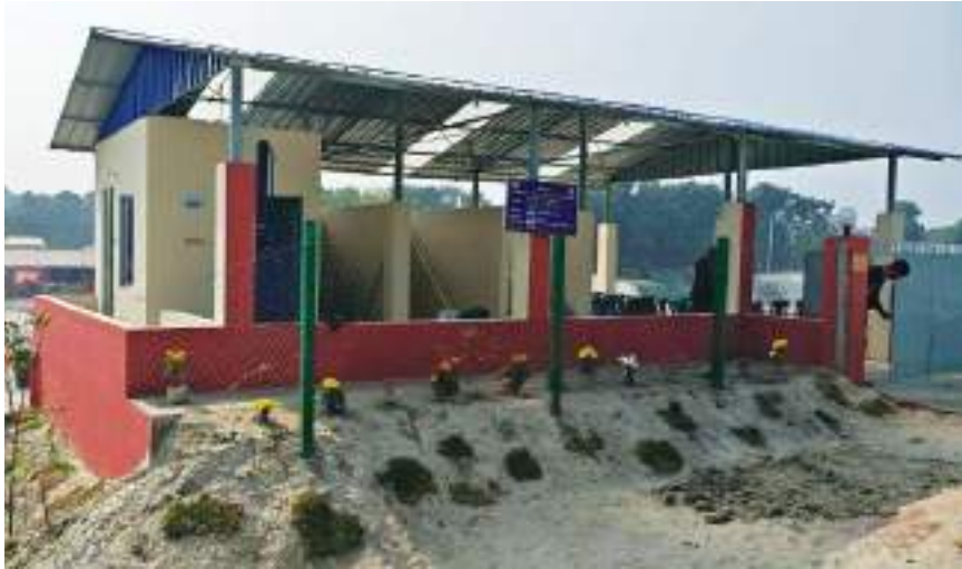
Figure 12: Material Recovery Facility (MRF) in Gorai Badh, Ward 10
